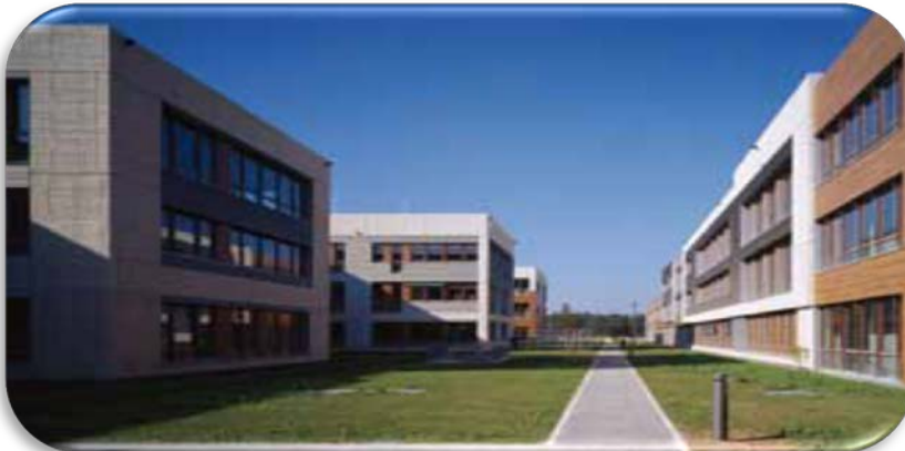
Group headquarters reduces the cost of electricity for lighting through automatic KNX controls
