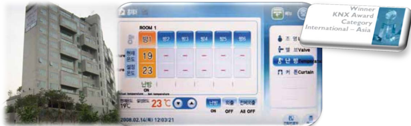
World standard in uniform design for apartment building in Seoul. Comfortable operation of KNX functions by a central touch panel: for example, menus for heating, curtains and lighting.
