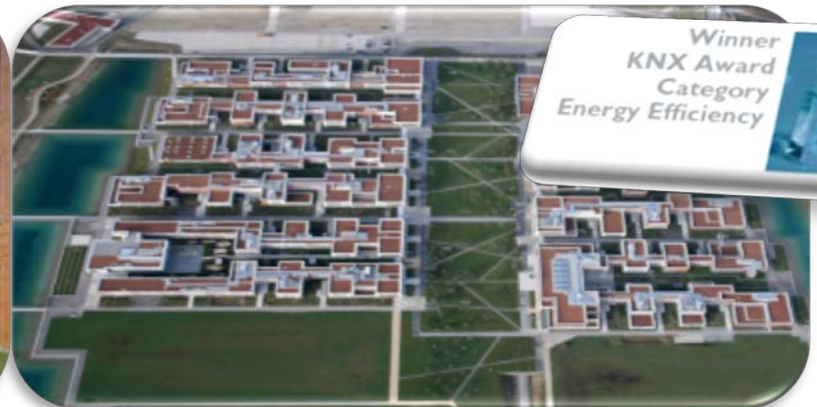
Six servers link the KNX 'worlds' in accordance with the building zones for lighting management.
